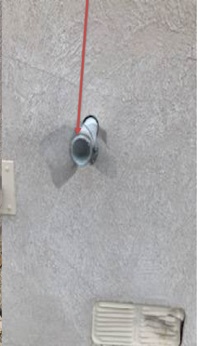
New screen replaced
