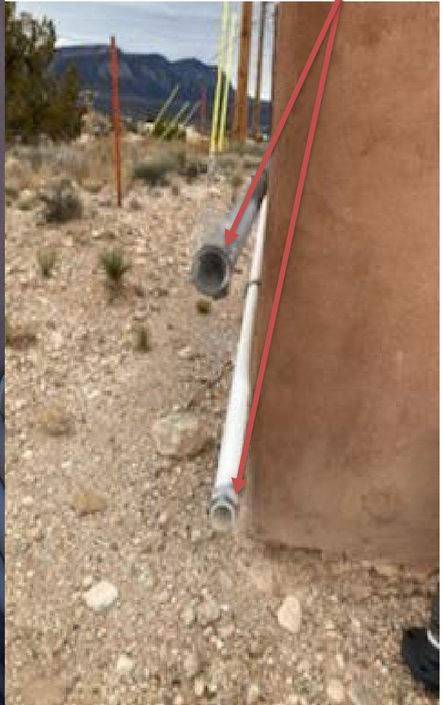
Screens have been replaced and added.
