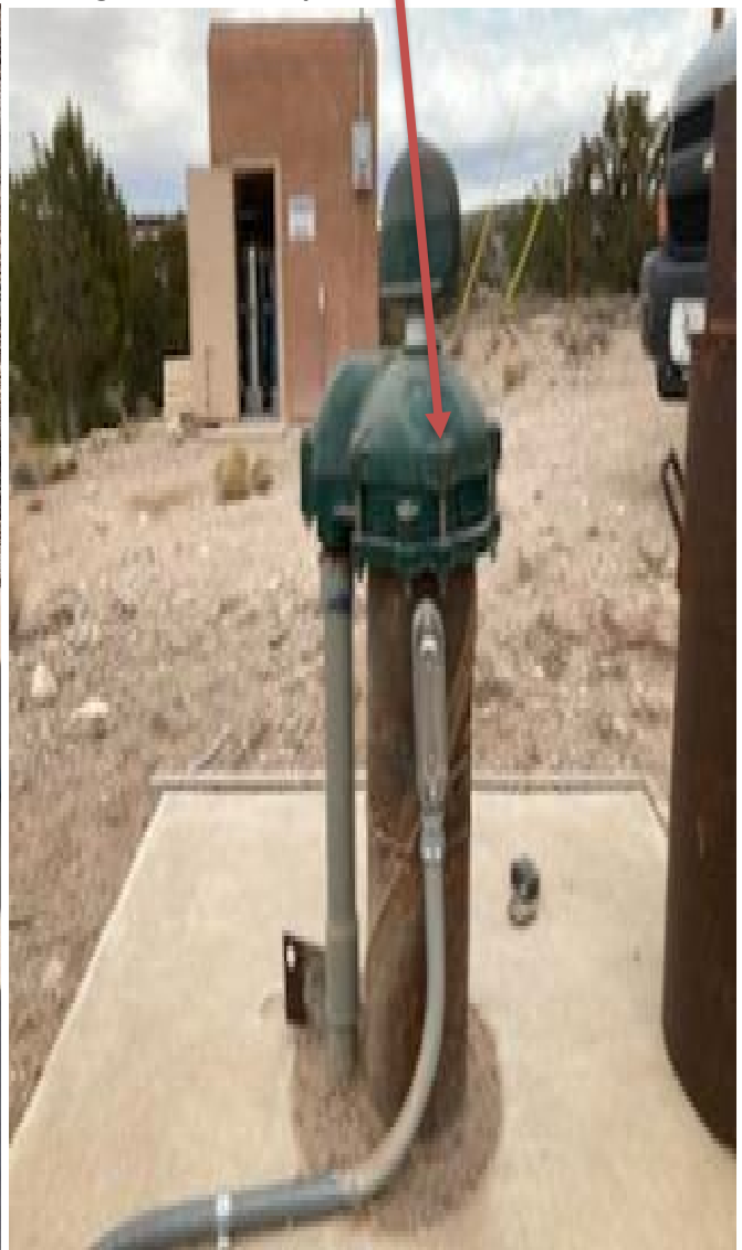
Bolts tighten and or replaced
