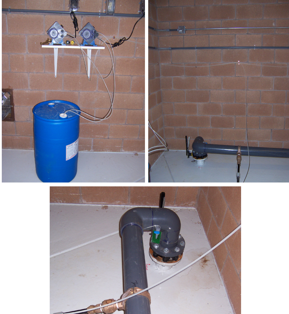
Figure 4-8. Chlorination Feed System
