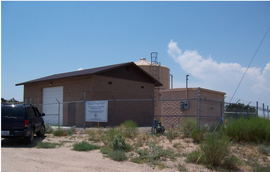
Figure 4-12. Nambé Pueblo Treatment Plant Building (Top: Building under construction; Bottom: Completed building)
