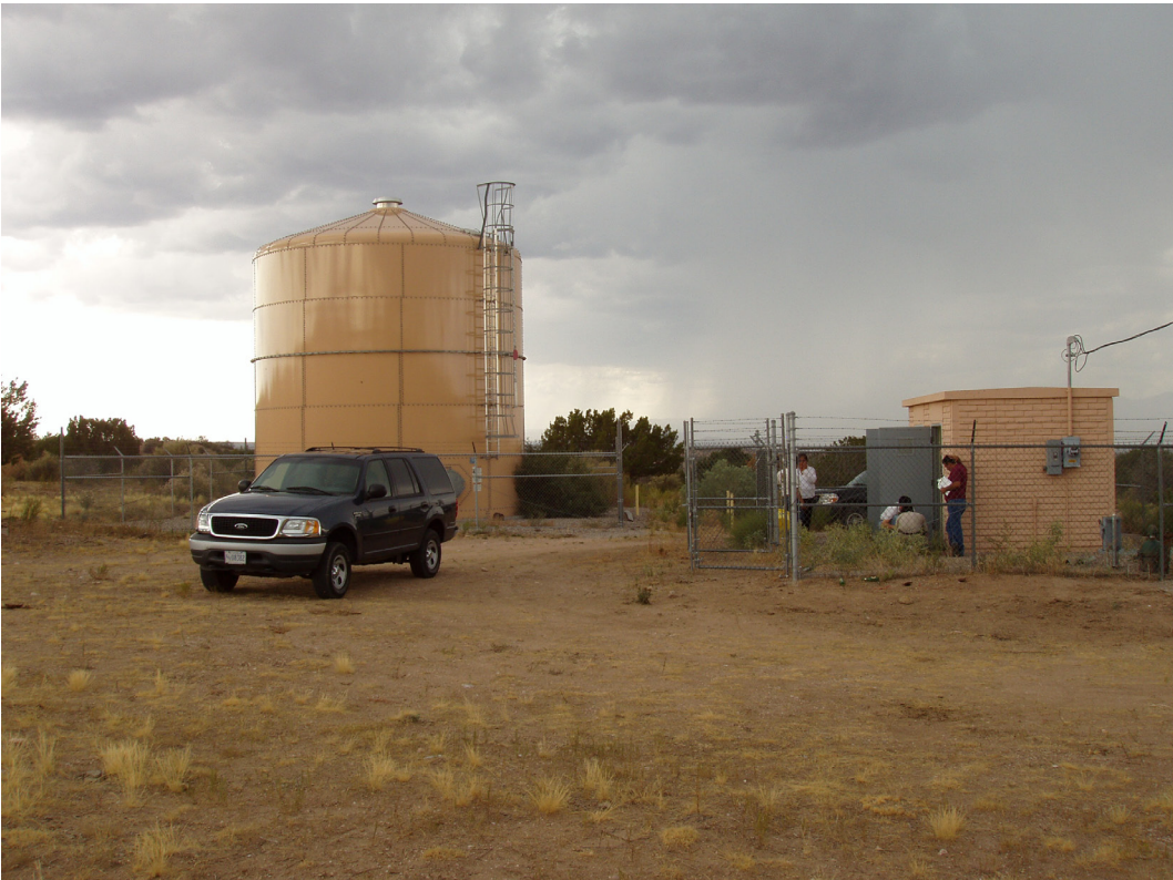
Figure 4-3. Pre-existing Pump House and Water Storage Tank
